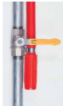
Hose nozzle interlock
